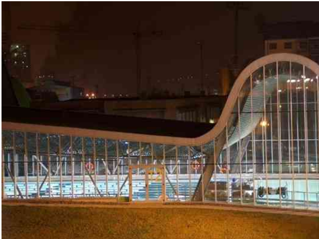
FACHADA PRINCIPAL NOCTURNA
