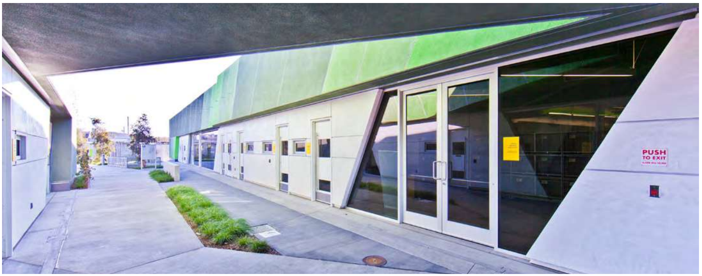
Imagen 22. Galería central South L.A. Animal Care Center and Community Center. Fuente: http://www.archdaily.com/407296/south-los-angeles-animal-care-center-and-community-center/51f28e85e8e44ea5b70001c3-south-los-angeles-animal-care-center-and-community-center-photo
