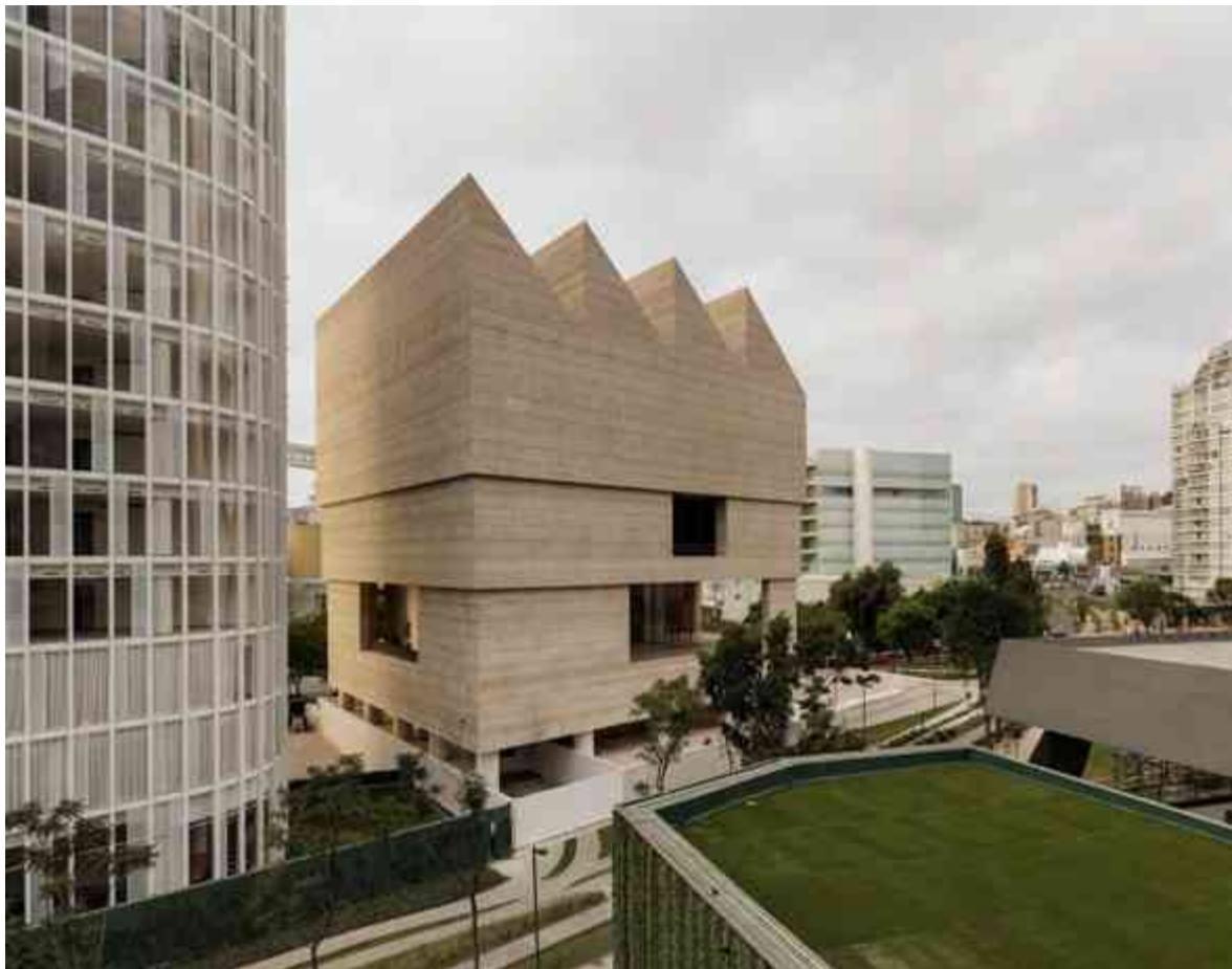
Imágen 15. Perspectiva Exterior. http://www.archdaily.mx/mx/768384/museo-jumex-david-chipperfield-architects/5578e503e58eced6280000a6-museo-jumex-david-chipperfield-architects-photo
