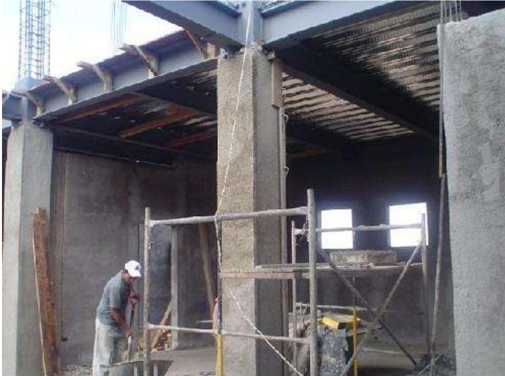
IMAGEN 63: AGUAS CALIENTES. COLUMNAS DE CONCRETO Y VIGAS (I.P.R) FUENTE:
