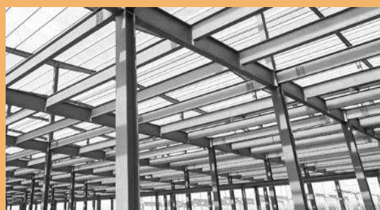
FIGURA 48: “Columnas de acero”, [Fuente: autodesk], en: https://www.autodesk.com/solutions/bim/structural-engineering
