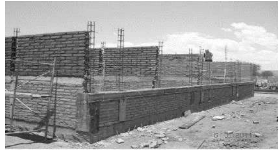
FIGURA 51: “Dalas de concreto armado”, [Fuente: Mel-construction], http://mel-construction.com
