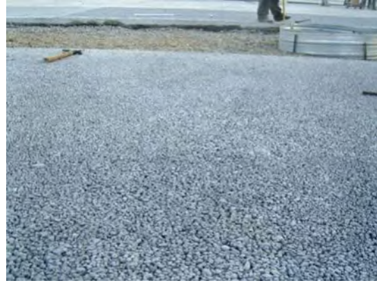
Fig. 76: concreto permeable.
