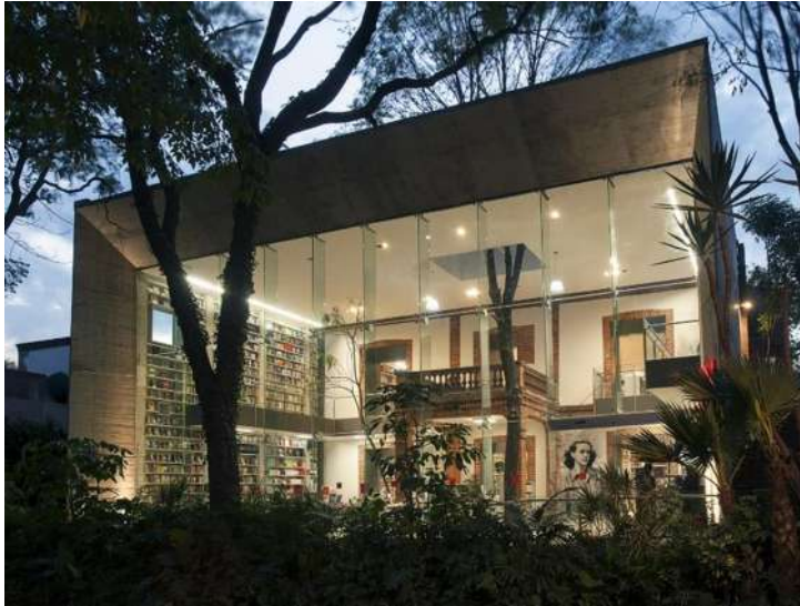
Ilustración 29. Fachada principal. Recuperado de: https://images.adsttc.com/media/images/5736/25e5/e58e/cecc/8d00/000d/large_jpg/CEEG_Entrance_AN_01.jpg?1463166417
