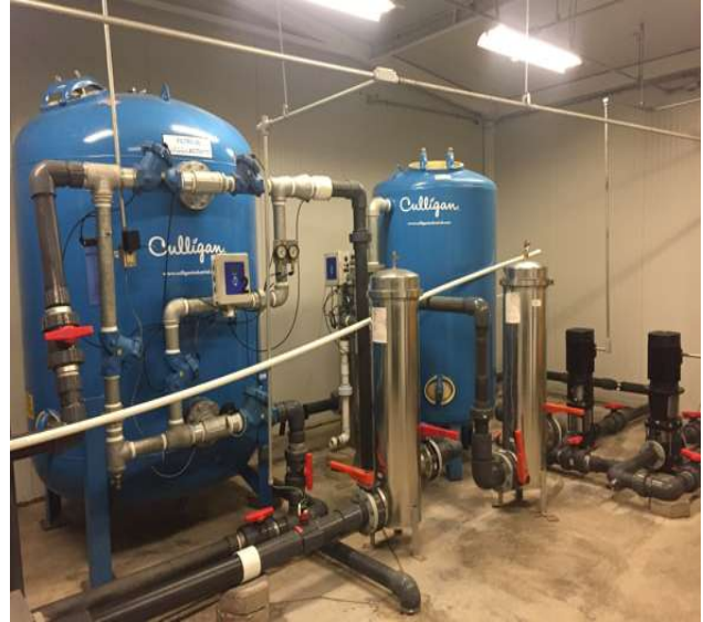
Figure 4.4: Left: sketch of a WCD of HAWC. Due to water's refraction index and its low cost, water is employed to fill in the WCDs [146]. Right: HAWC's site counts with a continuous purifying water system, which prevents the presence of impurities, contaminants or microorganisms inside each WCD of the experiment. In the figure the purifying water system can be seen ( Image source: HAWC Collaboration ).
