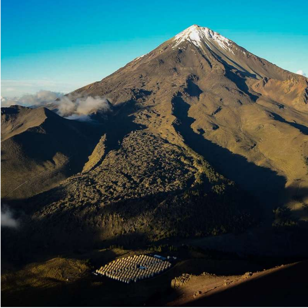
Figure 4.1: HAWC is an air shower detector designed to study the sky in gamma rays ( E = 100 \text{ GeV} - 100 \text{ TeV} ), and cosmic rays (up to 1 \text{ PeV} ). The experiment is located at 4100 \text{ m a.s.l.} (below the shower maximum, 640 \text{ g/cm}^2 ) on the slopes of the Pico de Orizaba Volcano in Puebla, Mexico. Thanks to its high altitude, HAWC can measure air showers with energies as low as 100 \text{ GeV} ( Image source: HAWC collaboration ).
