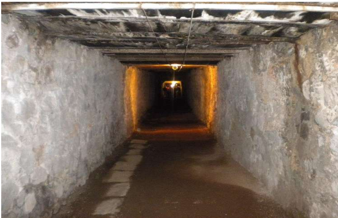
INTERIOR DEL SOCAVON PRINCIPAL
