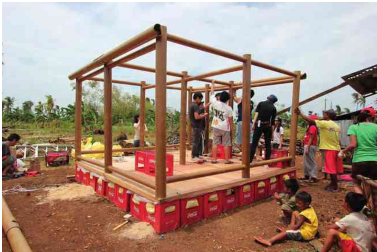
FIG. 70 "Paper Log House", Filipinas, 2014. Tomado de: http://www.shigerubanarchitects.com/works/2014_PaperEmergencyShelter-Philippines/index.html
