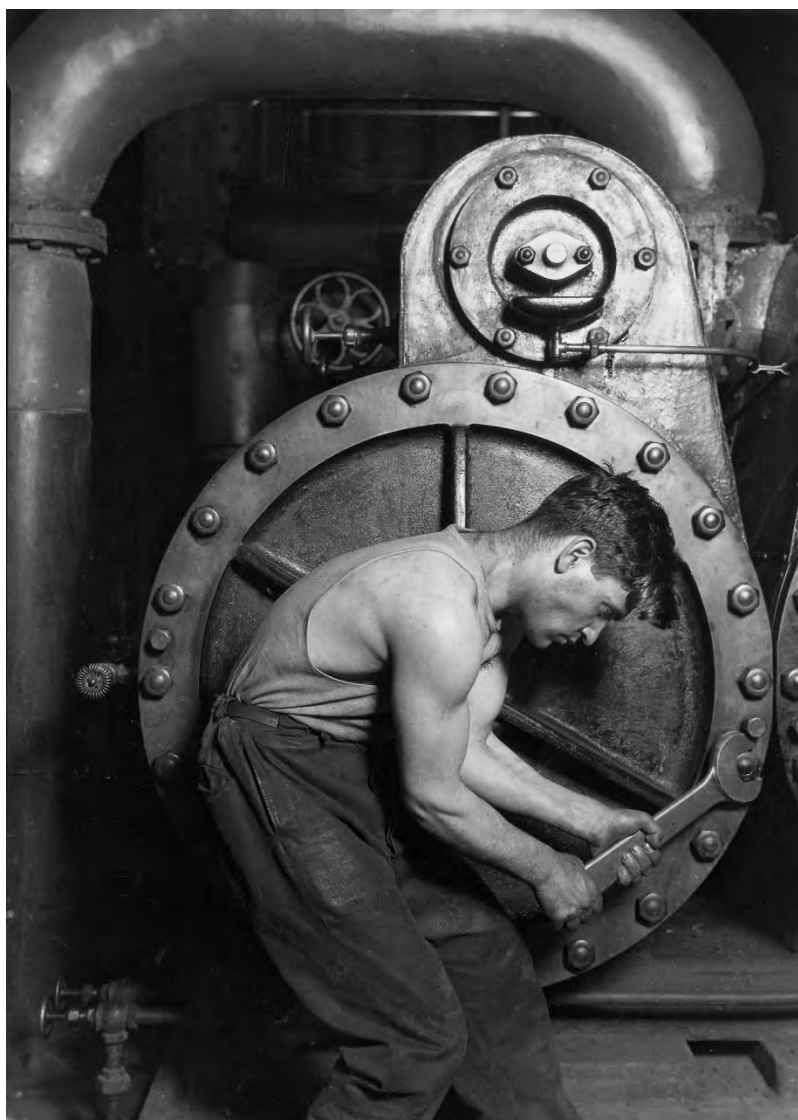
Fig. 20 Hine, L. (1920). Power house mechanic working on steam pump. Brooklyn Museum.
