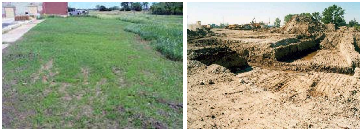
Figure 2- 19: Excavation of a site contaminated by metals, explosives, volatiles and semi-volatiles; soil before (left) and after (right) clean up.
