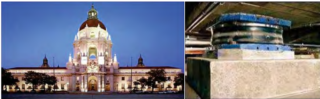
Figura 1.4.2 Pasadena City Hall en California U.S. ( http://www.earthquakeprotection.com/building_pasadena_city_hall_retrofit.html )
