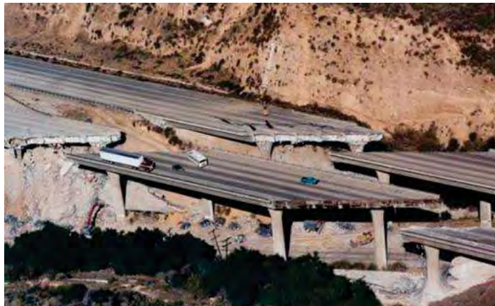
Figura 1.14 Puente Gavin Canyon dañado por el sismo de Northridge (1994). ( http://transit-safety.volpe.dot.gov/security/SecurityInitiatives/Top20/1%20-%20Management%20and%20Accountability/7%20--%20Accountability%20for%20Security/Additional/Effects_of_Catastrophic_Events/HTML/effects.htm )
