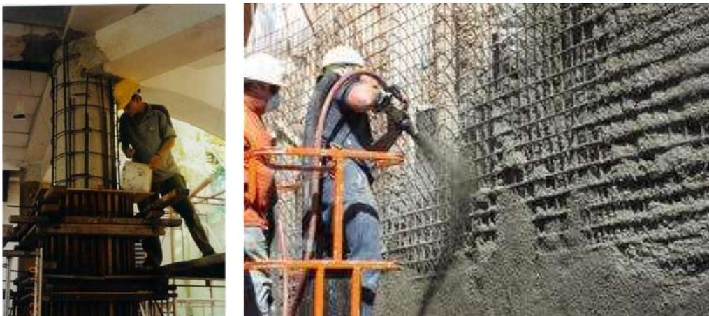
Figura 2.10 – Izquierda, encamisado convencional (*Brown Company*). Derecha, shotcrete ([http://t2.gstatic.com/images?q=tbn:ANd9GcSi7vxKmqrgDfjiB0wS6BEwCB0vJnKGG1tXIB0LtFDSPGSBGqA\\_](http://t2.gstatic.com/images?q=tbn:ANd9GcSi7vxKmqrgDfjiB0wS6BEwCB0vJnKGG1tXIB0LtFDSPGSBGqA_))
