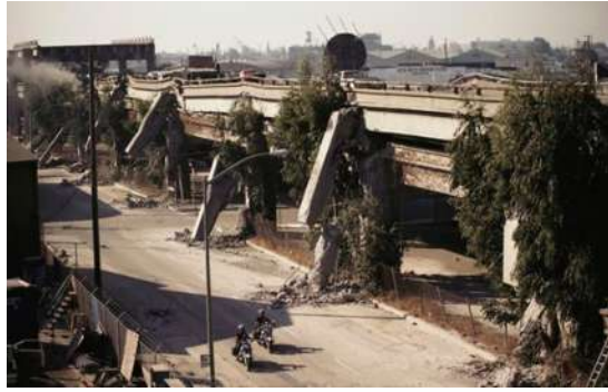
Figura 1.5 Freeway Cypress, Oakland, CA.
