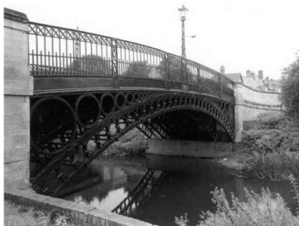
Figura 2.8 Puente Tickford. Tomada de: Hollaway L.C. and Cadei J., 2002.
