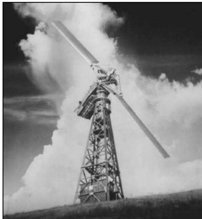
Figura 8. Turbina Smith–Putnam de 1250 kW [23].
