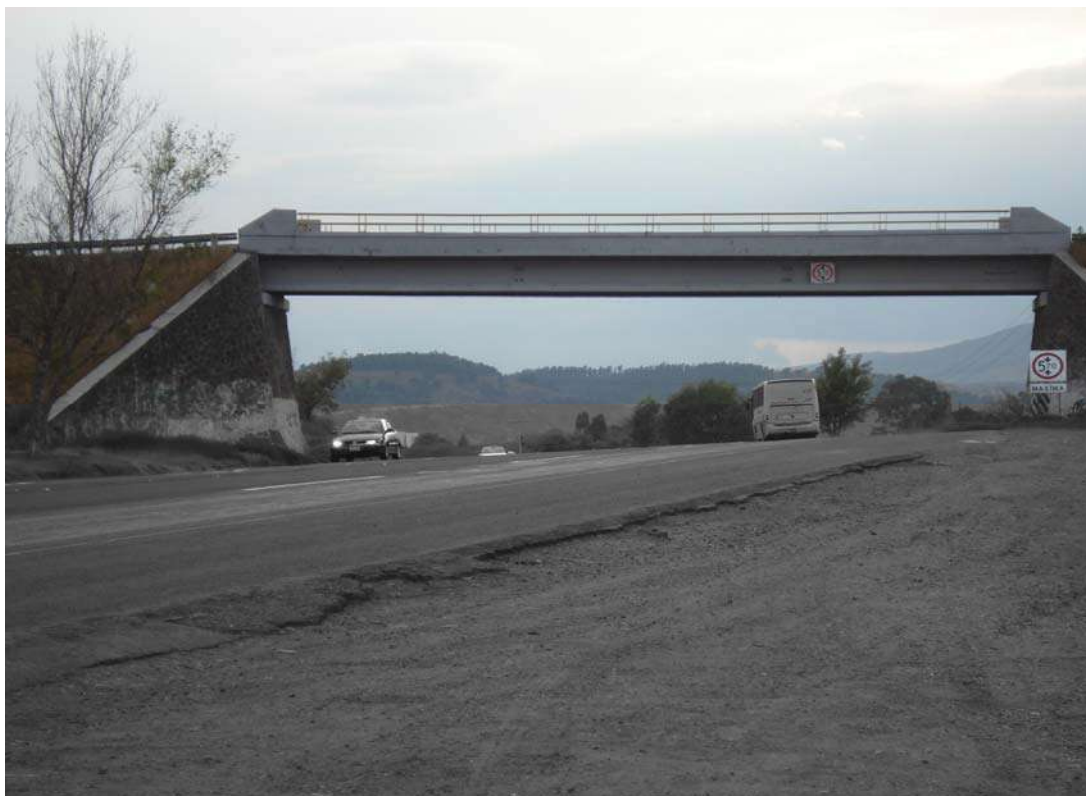
Figura 1.1 Paso Inferior Vehicular (PIV)
