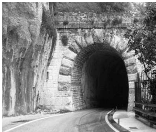
Figura 2.1 Entrada al túnel Furlo http://tectonicablog.com/wp-content/uploads/2011/09/Furlo_Tunnel_South.jpg25/01/2016 .
