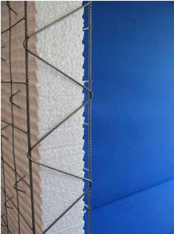
Figura 8- panel estructura QUALYPANEL COVINTEC ® 2",3" y 4"
