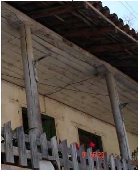
**IMAGEN No. 12 DETALLE DE APOYOS AISLADOS.**
