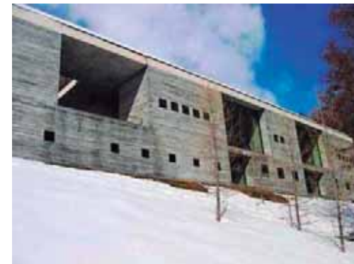
Thermes Vals Hotel, Switzerland Arquitecto: Peter Zumthor
