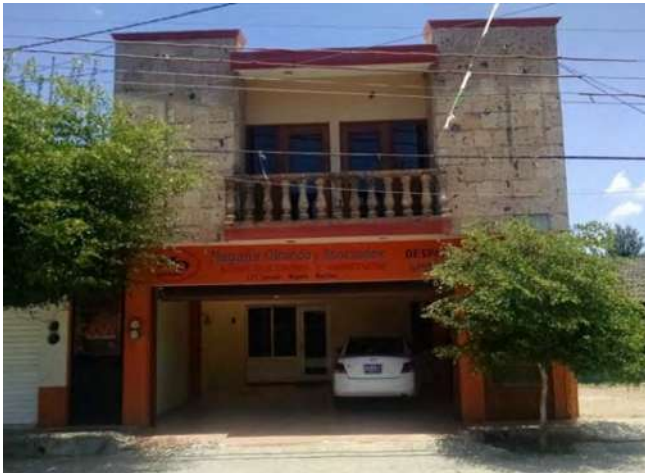
VISTA FRONTAL EXTERIOR
