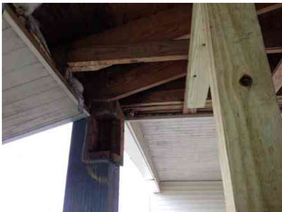
Fig. 71. Viga removida vista angular. Autor: JAPG.
