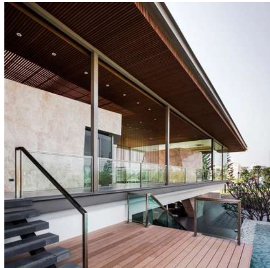
Ilustración 51. Clubhouse Gran Pinklao / Office AT.Bangkok, Tailandia. 2013. http://www.archdaily.mx/mx/02-344917/clubhouse-gran-pinklao-office-at
