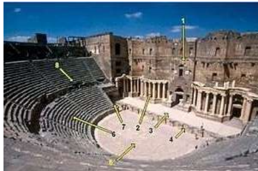
1. Scaenae frons 2. Porticus post scaenam 3. Pulpitum 4. Proscenium 5. Orchestra 6. Cavea 7. Aditus maximus 8. Vomitorium, Teatro Romano de Bosra, Siria.
