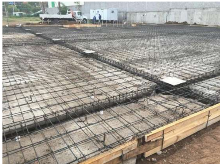
Fig. 63 [ https://mx.habcdn.com/photos/project/medium/armado-de-losa-de-cimentacion-270566.jpg ] FECHA DE CONSULTA: NOV/18]
