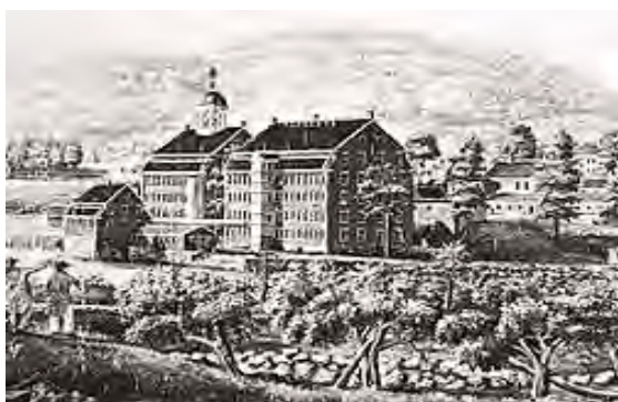
FIG. 4: Nave industrial, Boston manufacturing. FUENTE: Charles river museum AUTOR: MRJ.
