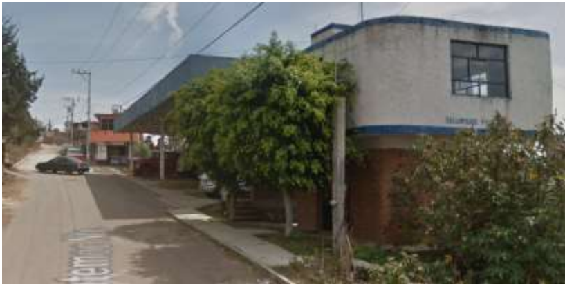
fig.39: fachada norte de la central de bomberos ciudad hidalgo, fuente: Fire station. 2020. Fire Station. [Online] Available at: < https://www.google.com/maps/place/Estaci%C3%B3n+De+Bomberos/@19.7060669,-100.5536097,118m/data=!3m1!1e3!4m5!3m4!1s0x85d2cbbf9f349a5b:0xe4e0e9eccf84e590!8m2!3d19.7061715!4d-100.5534109 > [Accessed 15 October 2020].
