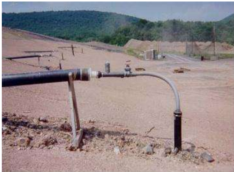
Figura 4-3 Colector horizontal.
