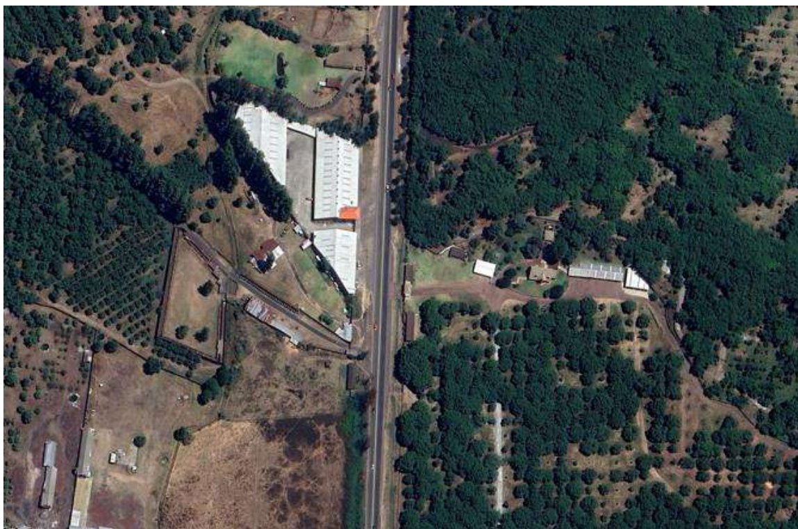
Figura 3-1. Carretera MEX-037 “Carapan – Playa Azul”, tramo “Carapan – Uruapan”, km 8+300
