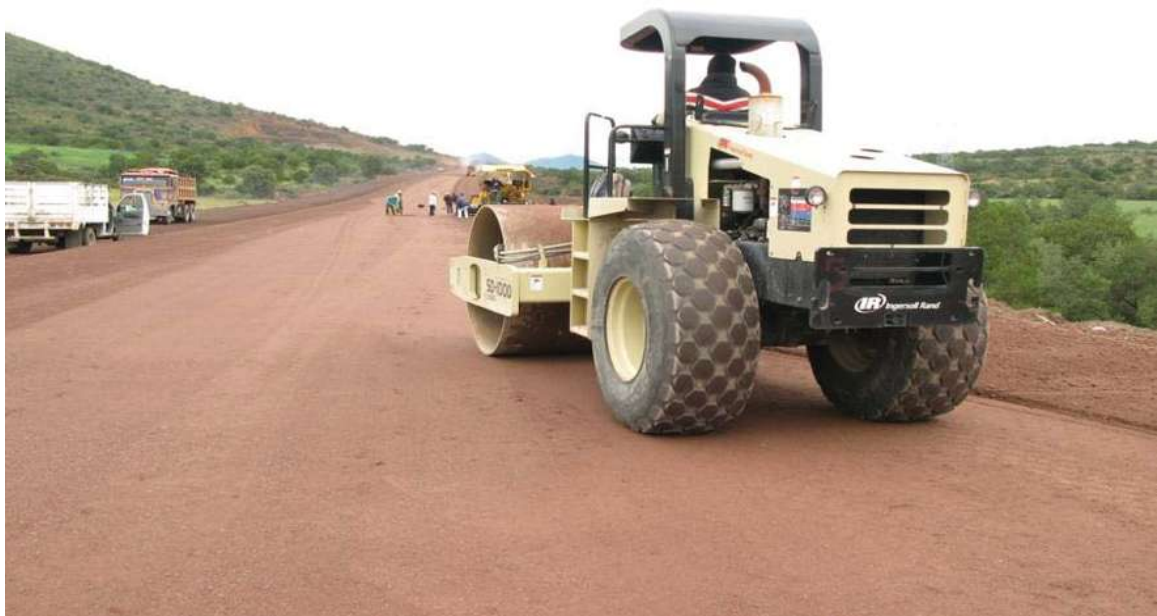
COMPACTACION CAPA SUB-BASE
