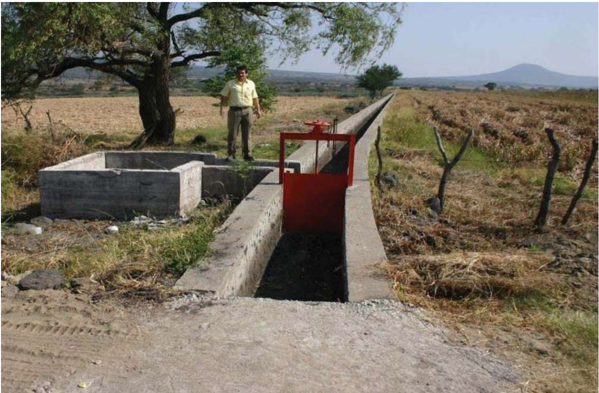
PRESA ING. JOSE ANTONIO TORRES CANAL PRINCIPAL Km I + 000
