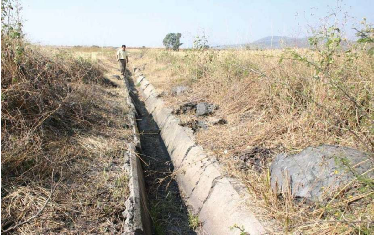
PRESA ING. JOSE ANTONIO TORRES CANAL PRINCIPAL Km 1+ 520
