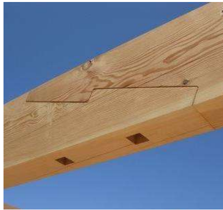
Imagen 72. Center post scarf in Timber Framing_Log construction.
