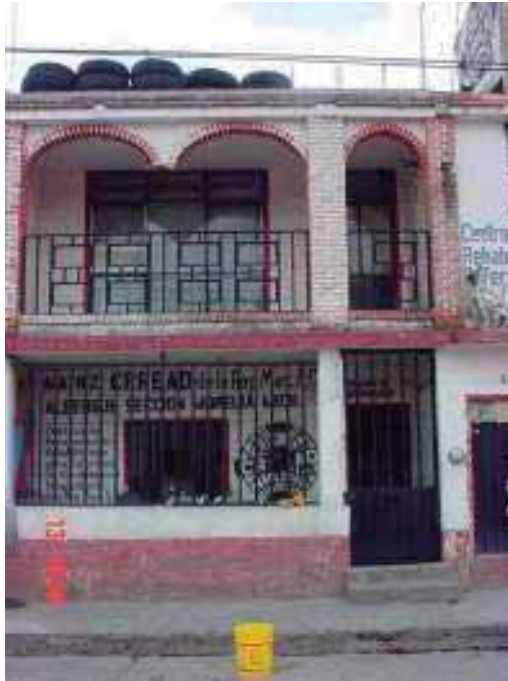
FACHADA PRINCIPAL DEL C RREAD
