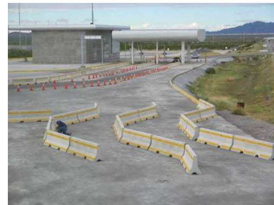
BARRERAS DE CONCRETO GARITA ADUANAL SAMALAYUCA, CHIHUAHUA
