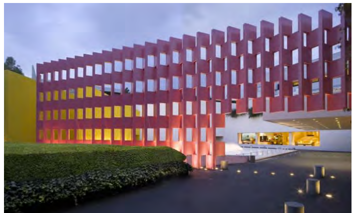
F69. Fachada Principal
