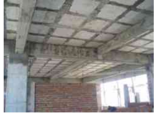
F58. Losa Reticular
