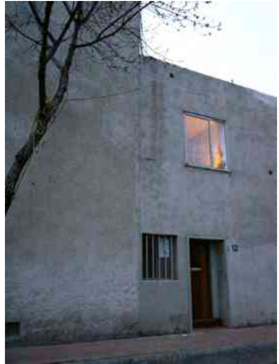
F70. Fachada Principal
